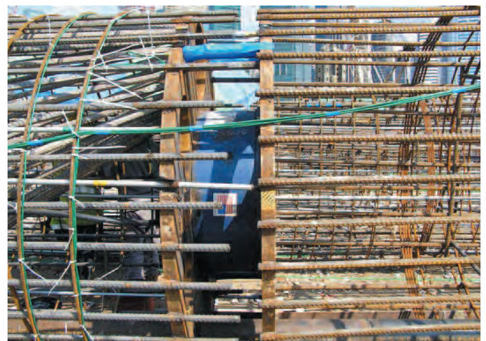
An O-cell setup assembled in a reinforcing cage.
