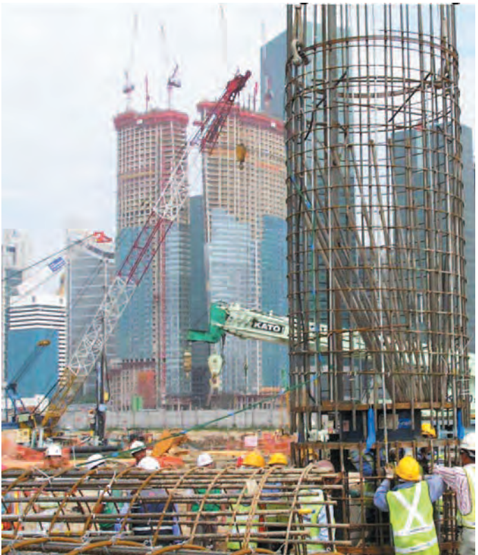
Installation of test shaft cage with O-Cell assembly.
