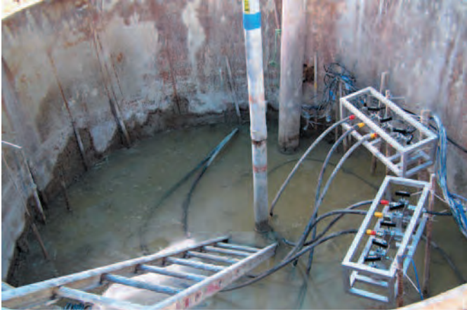
Strain gauge wiring and O-Cell hoses at the top of shaft.
