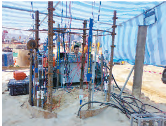
O-Cell testing in progress.
