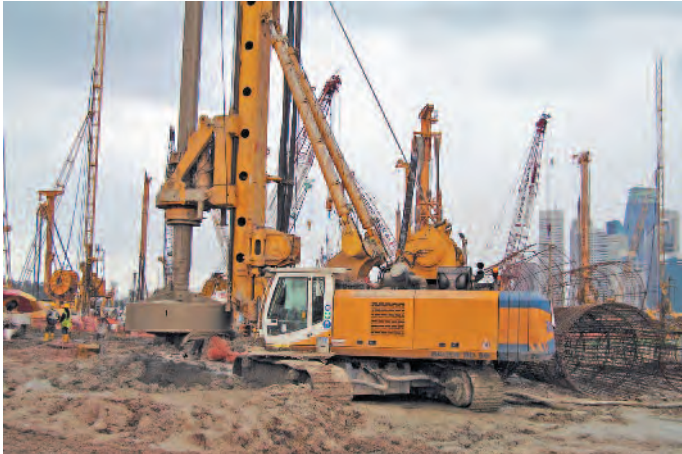
A drill rig excavating one of the test shafts.
