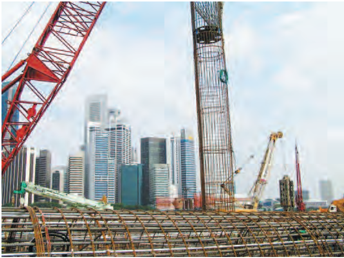
Lifting a test shaft cage with O-Cell assembly.
