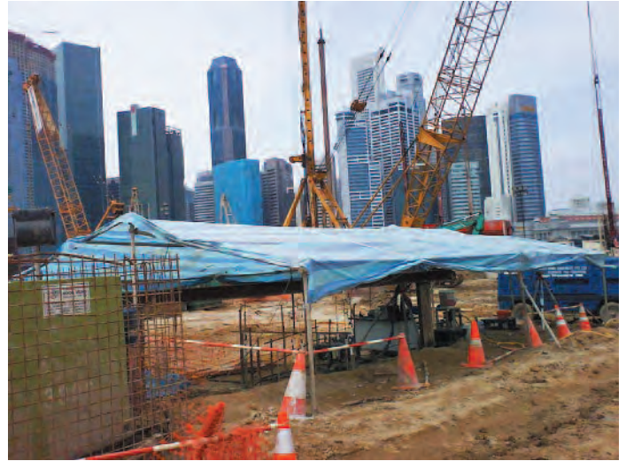
O-cell test setup; note the minimal logistical support required.
